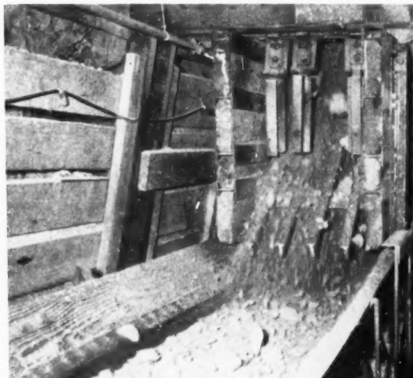
LEFT: In the new slusher-conveyor system developed at Miami Copper, ore is passed from the scraping level to the conveyors through a sloping grizzly that allows the fines to pass, padding the belt against the flow of coarser material. RIGHT: The Mexican set-up is here used by Pete Smith in developing the undercut level of a new block to be caved.
